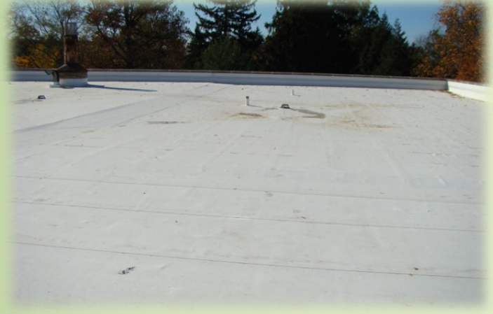
Moreau Hall new white roof
