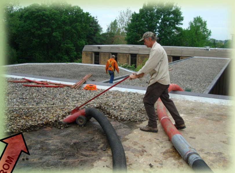
River rock being removed and salvaged off Madeleva Hall
