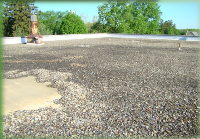
Moreau Hall old ballast roof
